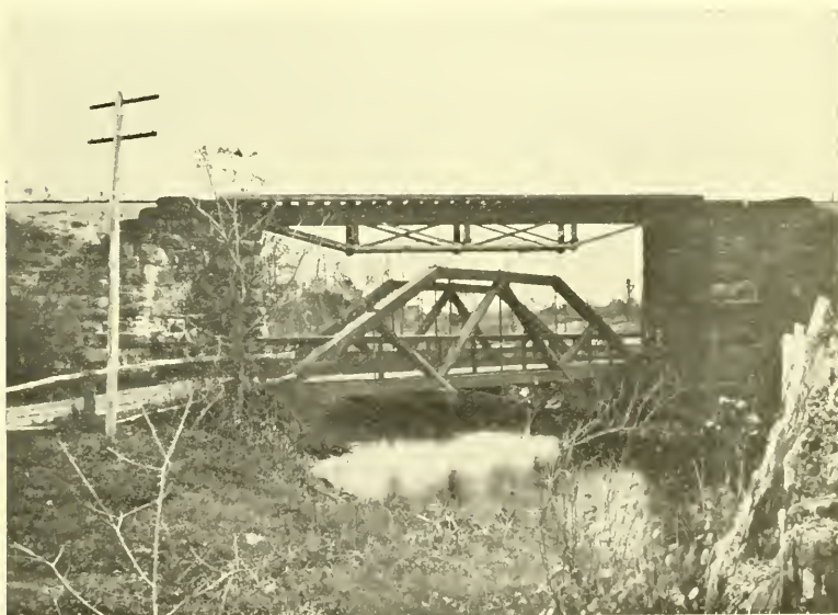
RAILROAD AND HIGHWAY BRIDGE OVER THE MUDDY RIVER.
